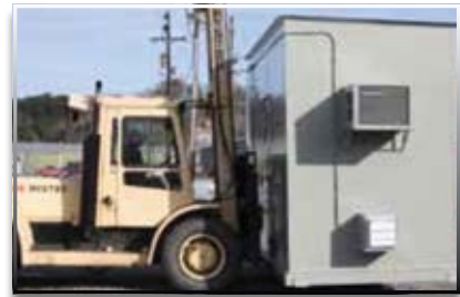
Building arrives on a tractor-trailer.
